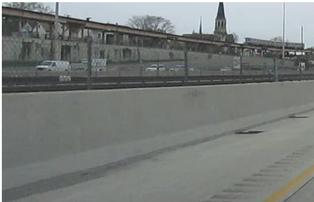
Figure 41. View of Barrier at Point of Impact [22]
