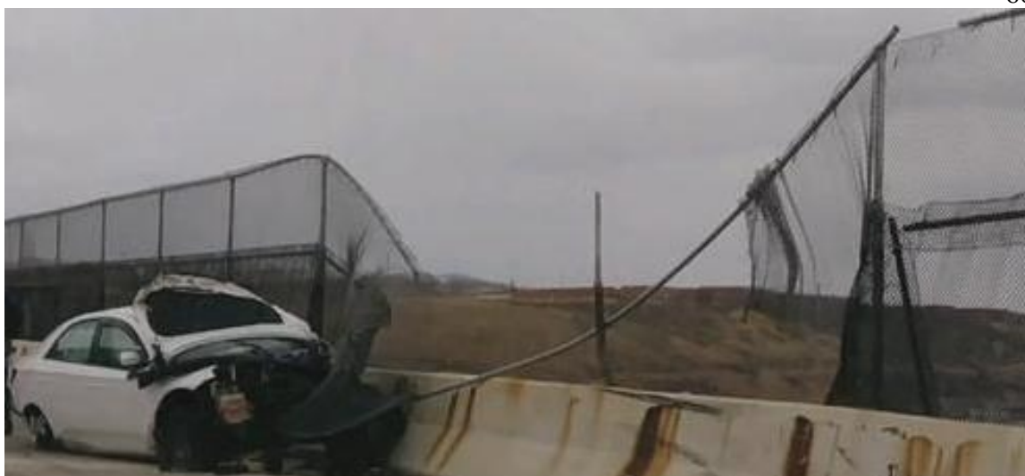
Figure 40. Valley View Vandal Protection Fence Crash [21]
