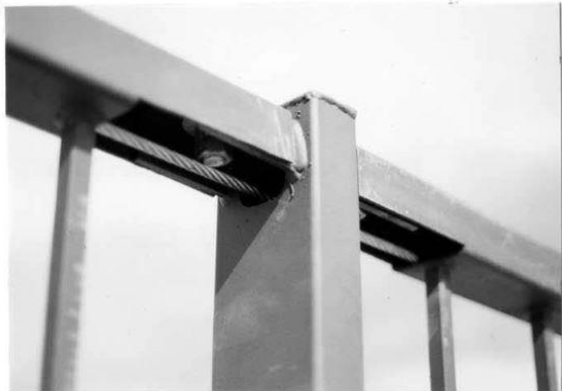
Figure 37. Tension Cable Taper and Rail Design
